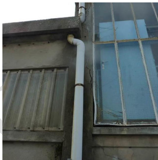
Figure 13 : Zédé - Fissures façade Nord
