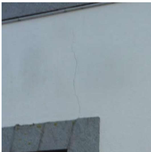
Figure 31 : Bât B - Fissure façade
