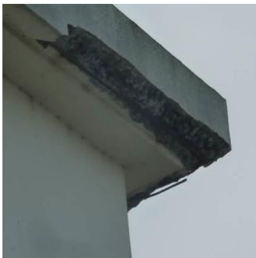
Figure 12 : Zédé - Epaufrure
